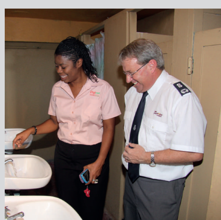
Eleen Rankine checks the pipes in the renovated bathrooms at the Salvation Army while John Williamson, Territorial Development Director, looks on.
